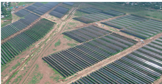
Meridional Solar SL Granja Solar Zambrano II
